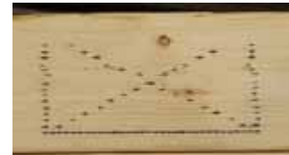
Figure A-12: Lateral Bracing Symbol
