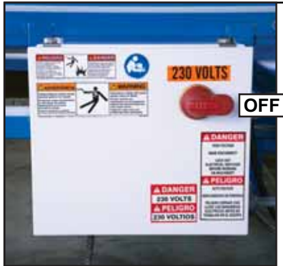
Figure 4-9: Lockout Mechanisms for Various Peripheral Components
